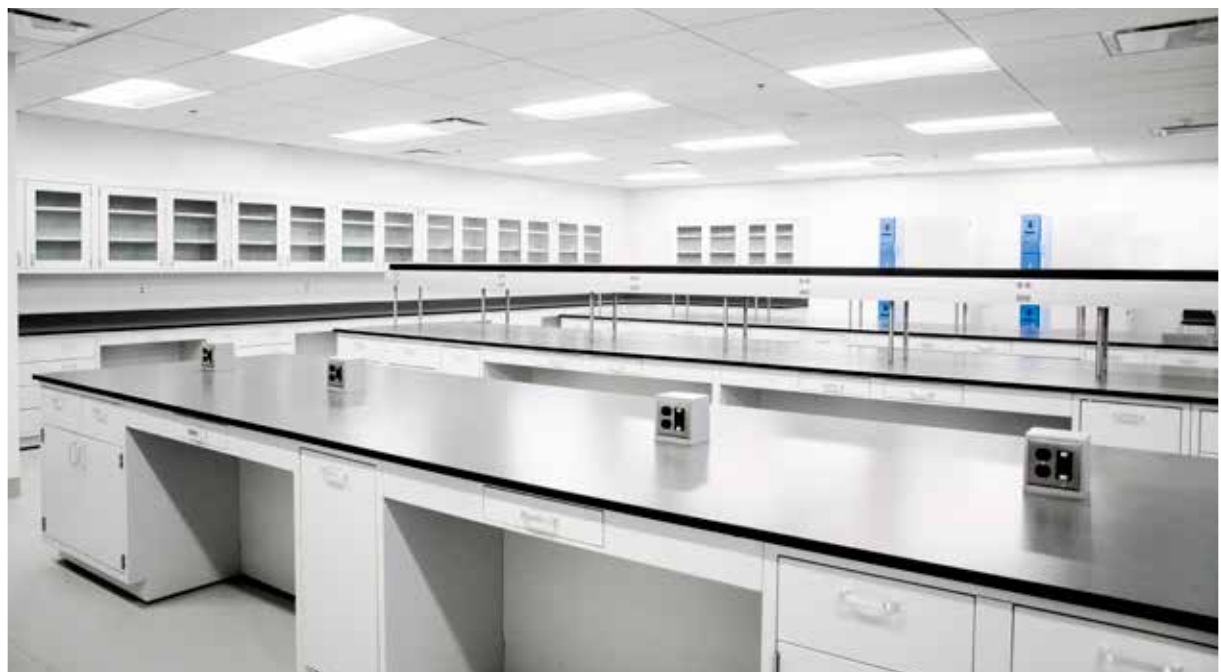
Built in lab steel lab furniture with acid resistant phenolic resin tops. Serious lab work completed here.
