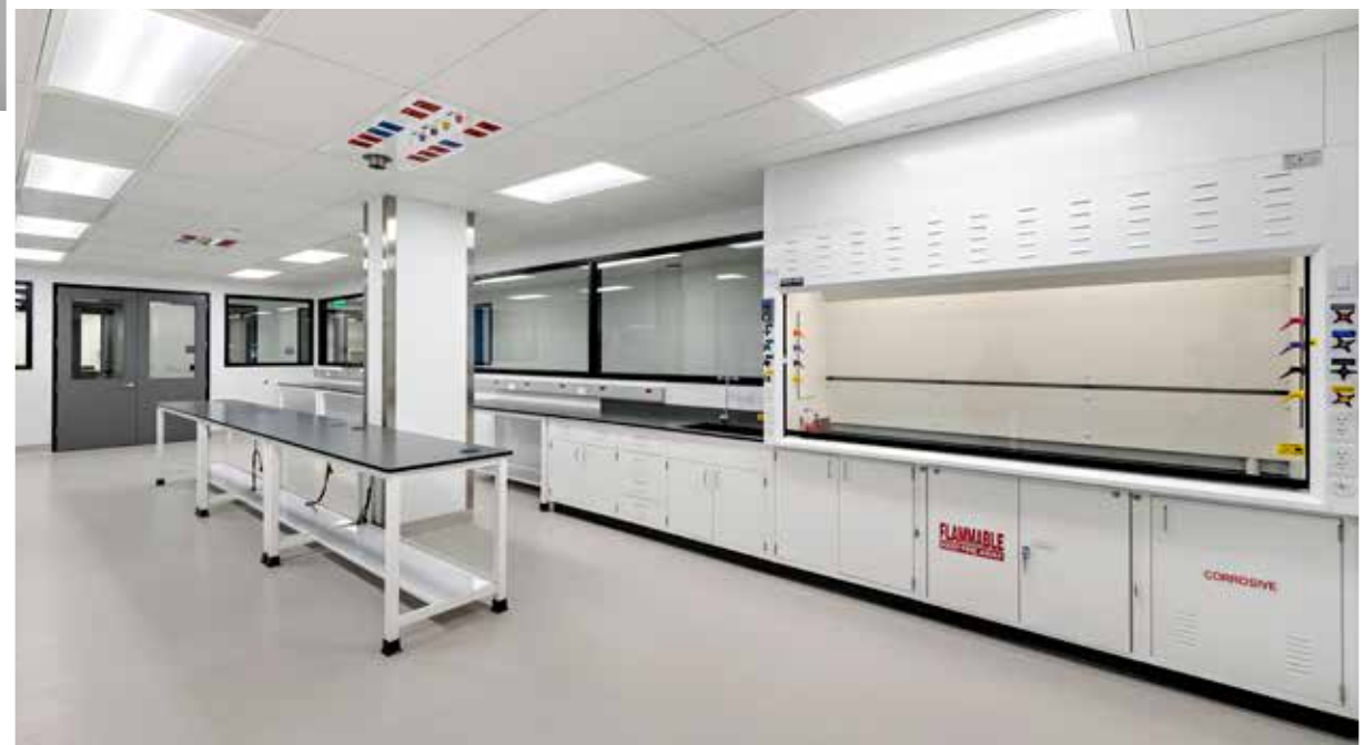
Floor mount/ walk in and bench top exhaust fume hoods. Timeless lab design.
